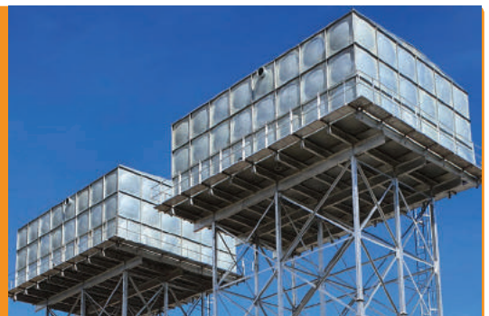
Water Tanks at Naivasha SEZ.
