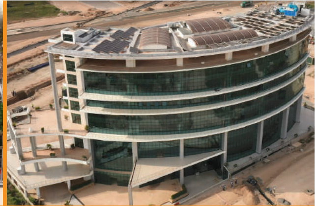
Konza Technopolis Head Office.
