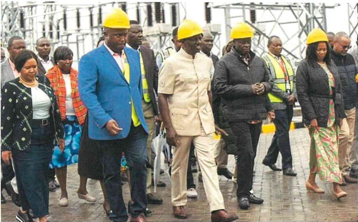
H.E. The President Dr. William Ruto inspecting the power sub-station at the Naivasha SEZ
