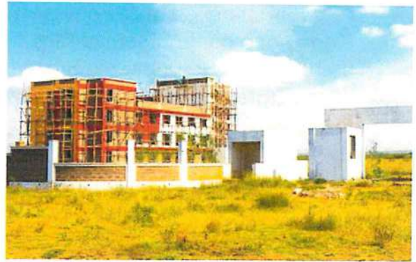
The gate under construction
