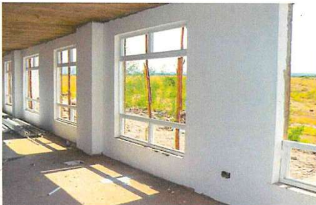
Ongoing fitting of windows
