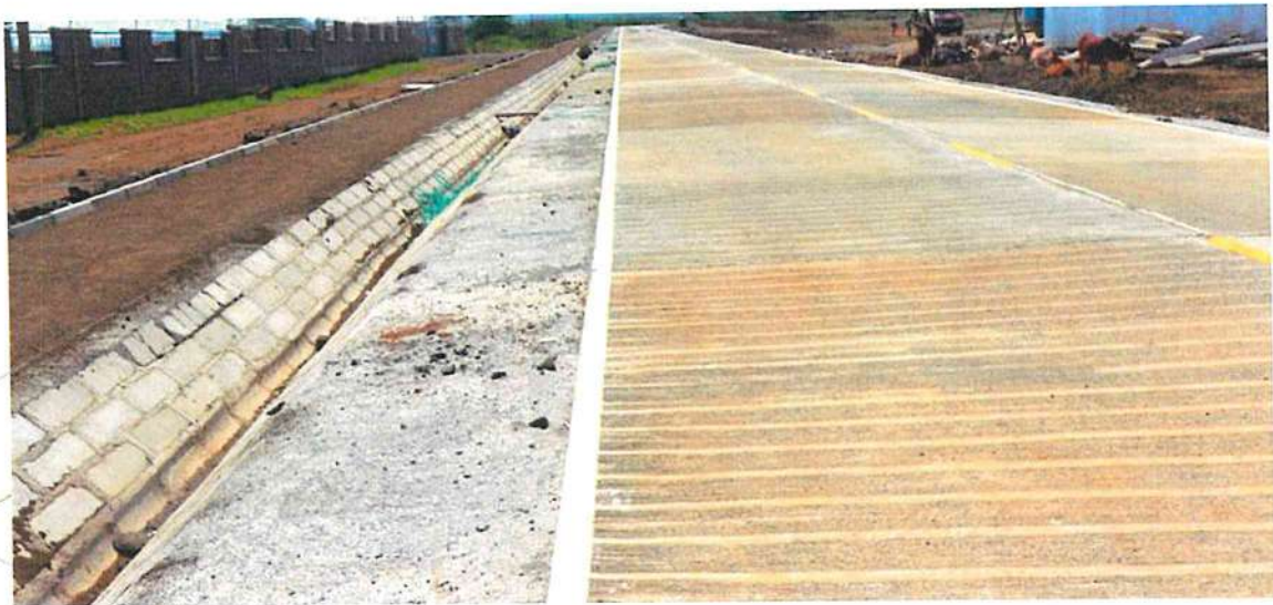
Completed Pedestrian footpath, side drain, shoulder and Concrete pavement
