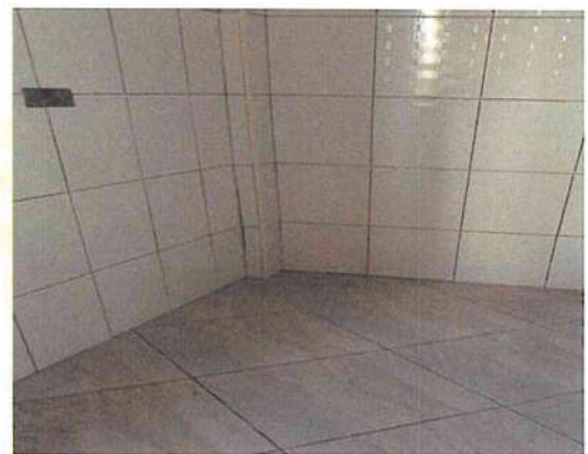
Ongoing tiling of internal common areas
