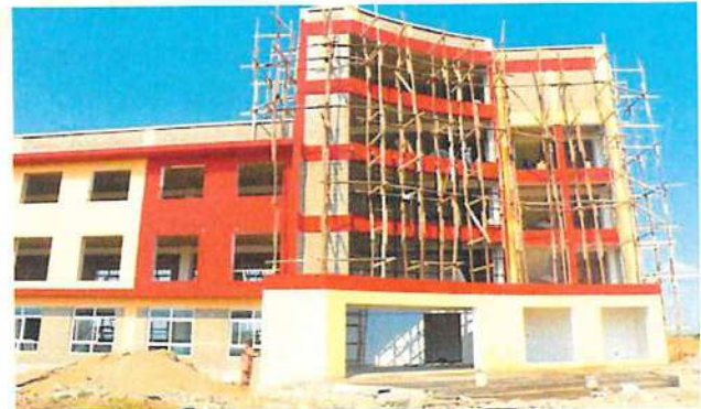
The One-Stop Shop/Administration Building under construction
