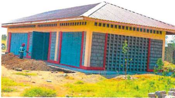
The Generator/Power house under construction
